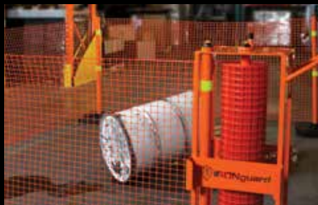
SECURE A TEMPORARY HAZARDOUS AREA
